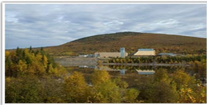
Mine Site Buildings and Mt. Pleasant
